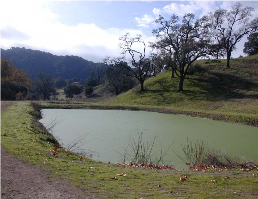
Figure 12: Wastewater Percolation Pond
