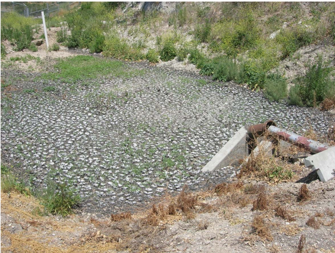
Figure 13: Sludge Drying Bed at the Lopez Lake Recreation Area Sewer Treatment Plant
