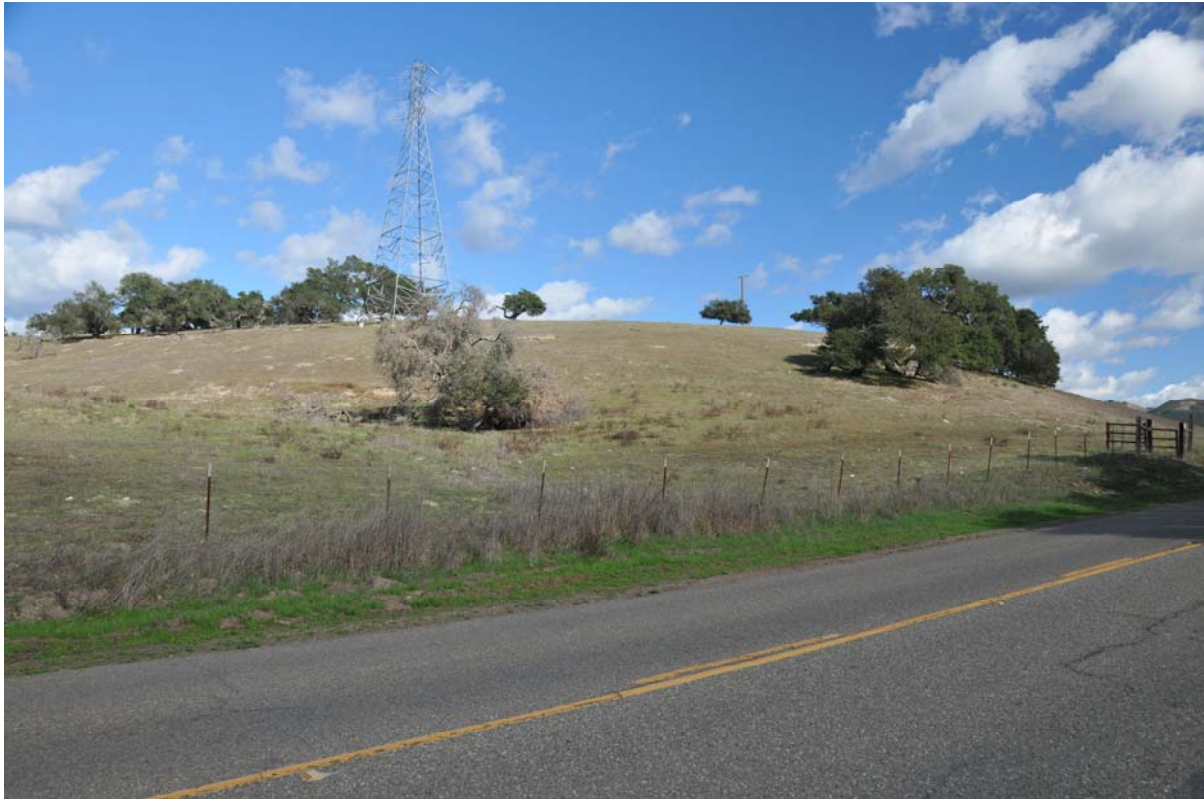
Figure 16: Terminal Reservoir Watershed Section Not Protected by Diversion Channel
