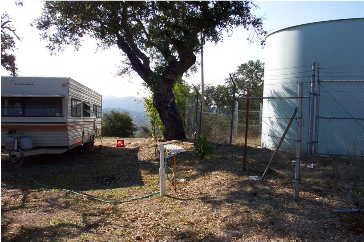
Figure 20: Private Property Near Domestic Tank
