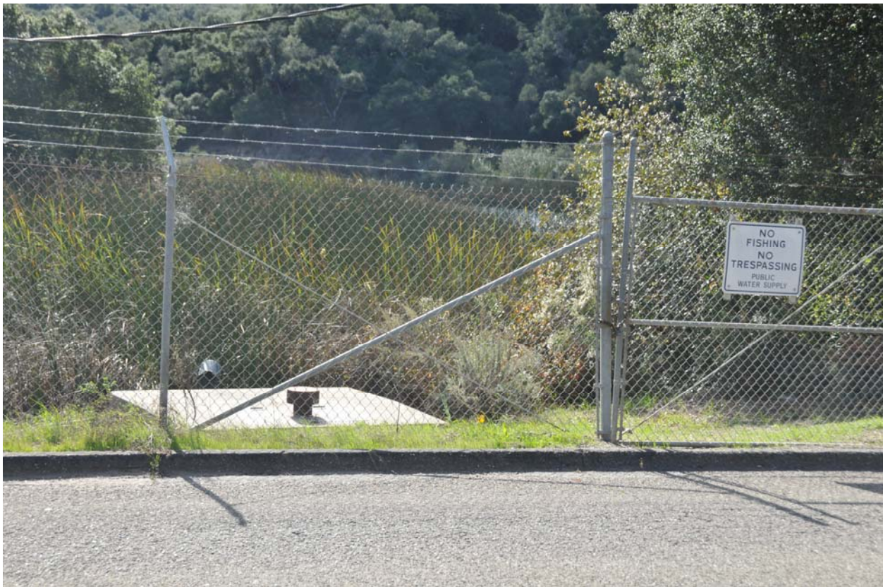
Figure 17: Terminal Reservoir Chain-link Fencing With Barbed Wire Top
