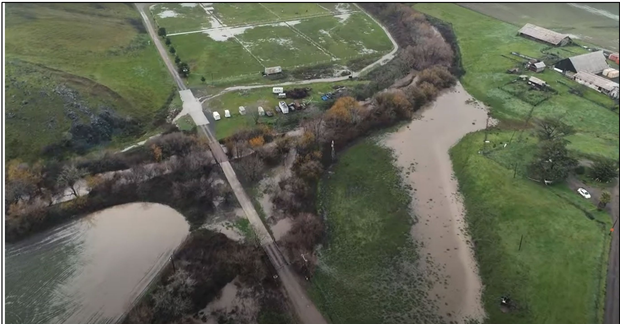
Figure 2 – January 2019 Downstream of Buckley Road
