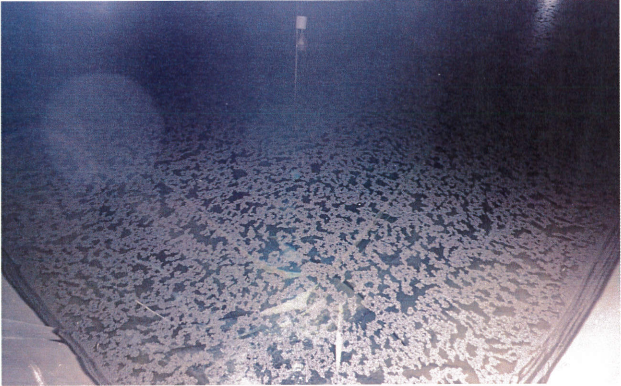
Photo 3: Interior of Reservoir 1
