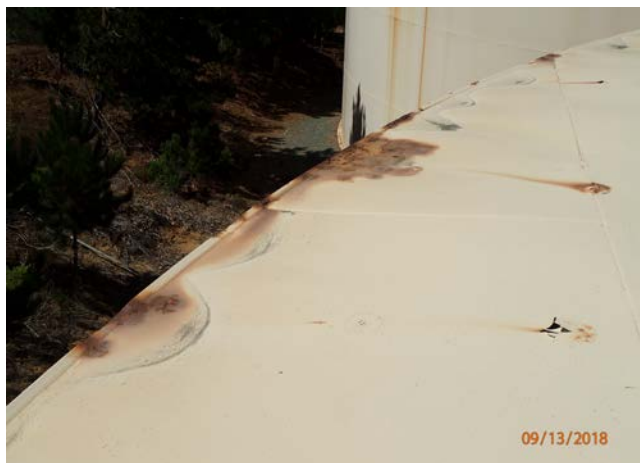
Figure 3 and 4 – Corrosion on roof at Kings Reservoirs.
