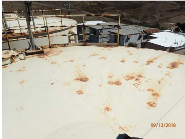
Figure 5 and 6 – Corrosion on roof of Blanca Reservoirs.
