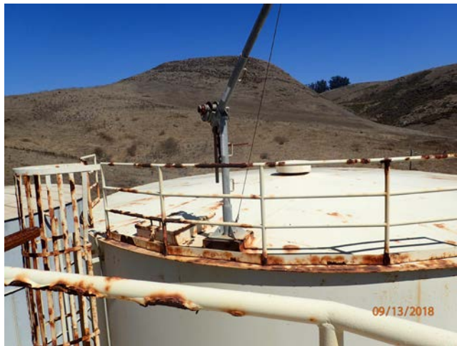
Figure 7 and 8 – Corrosion on Blanca Reservoir (left) and picture of exterior paint at Elena East Reservoir (right).
