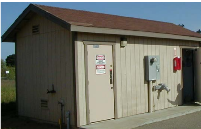
Source: Los Osos CSD South Bay Well House
