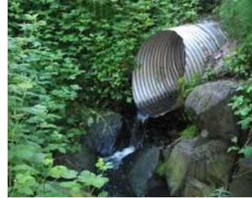
Point Source Discharge Pipeline
