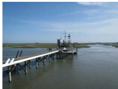
Automated Monitoring in Estuary
