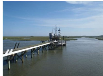
Automated Monitoring in Estuary
