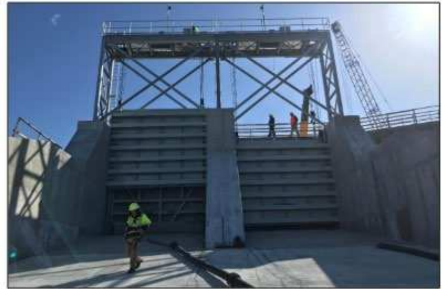
Upper Salmon Dam Gated Spillway
