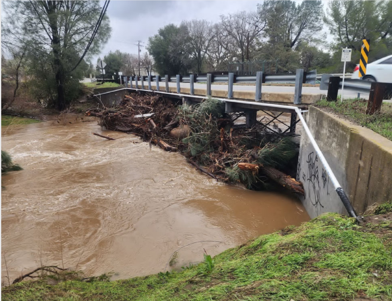
El Camino Real @ Santa Margarita Creek (County Public Works)
