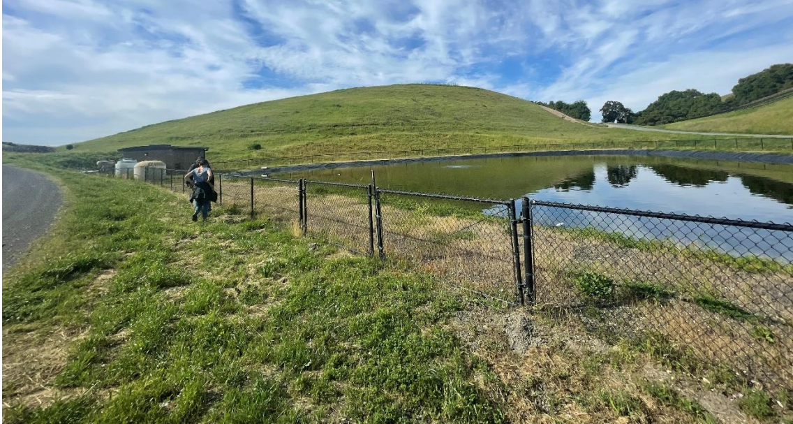
Photo 1. Pond connected to Pump house that feeds irrigation system.
