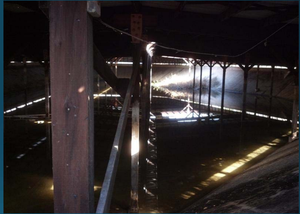
Existing Fox Hollow Reservoir, Interior
