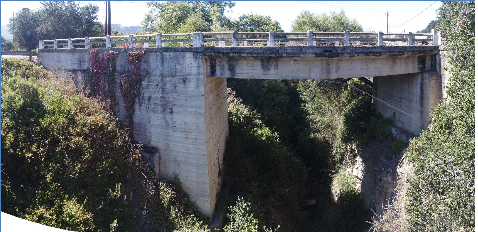
(e) Existing Huasna Road Bridge panorama looking north.
