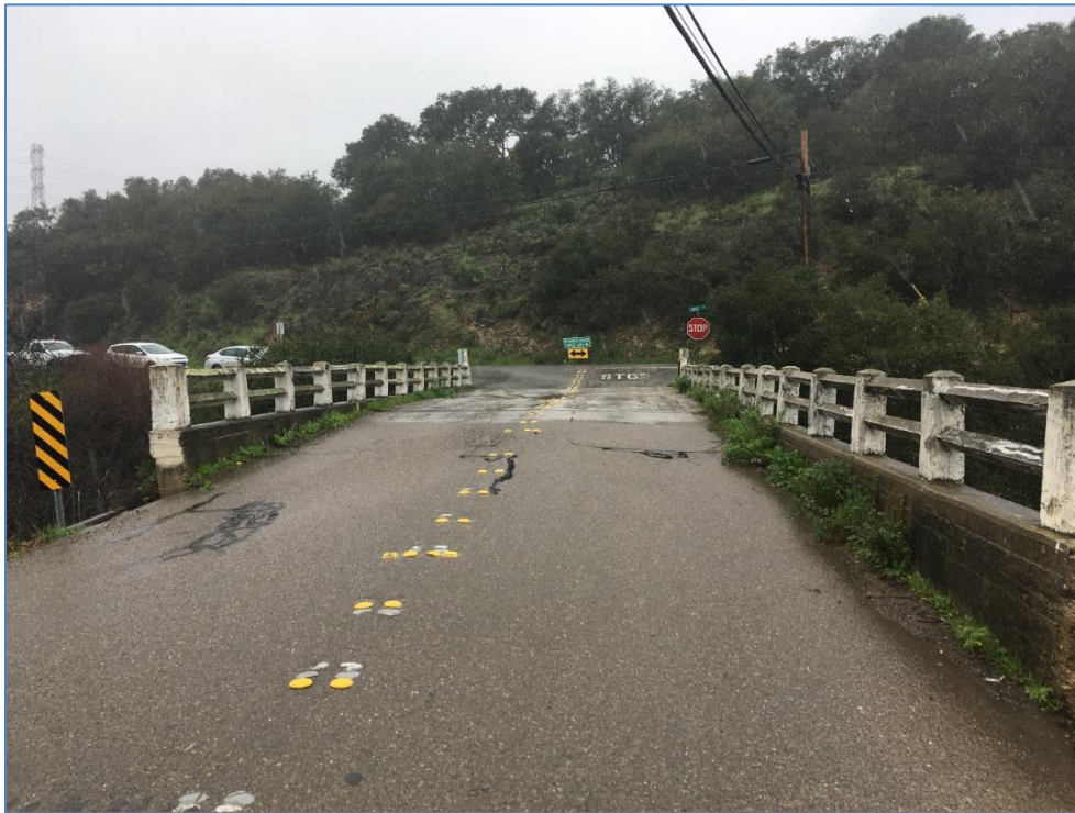
(b) Existing Huasna Road Bridge looking west to Lopez Drive.
