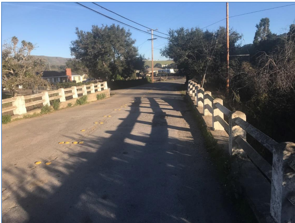
(c) Existing Huasna Road Bridge looking east along Huasna Road.
