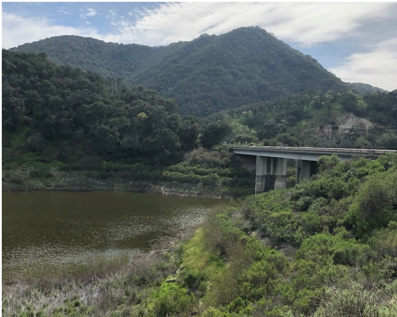
Figure 2. Lopez Drive Bridge
