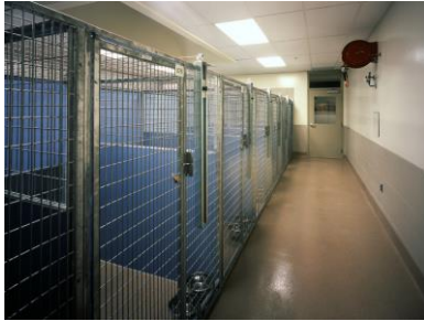
Typical Dog Ward with prefabricated kennels, epoxy resin floors and wall mounted cleaning system
