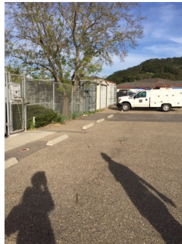
Exterior Storage and Parking
