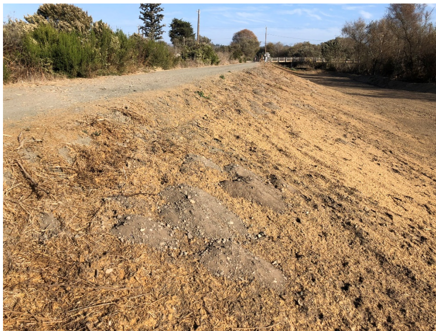
Figure 3: Rodent Burrows on north levee interior slope (facing east; 22 nd Street Bridge in background)
