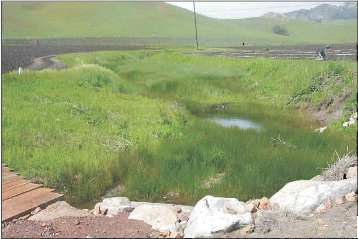
Photograph 39: View of middle reach of drainage T-1 at an existing culvert and driveway for the Tonini property, facing upstream and north. Note vernal marsh habitat within the drainage bounded by active agricultural land within the adjacent uplands.
