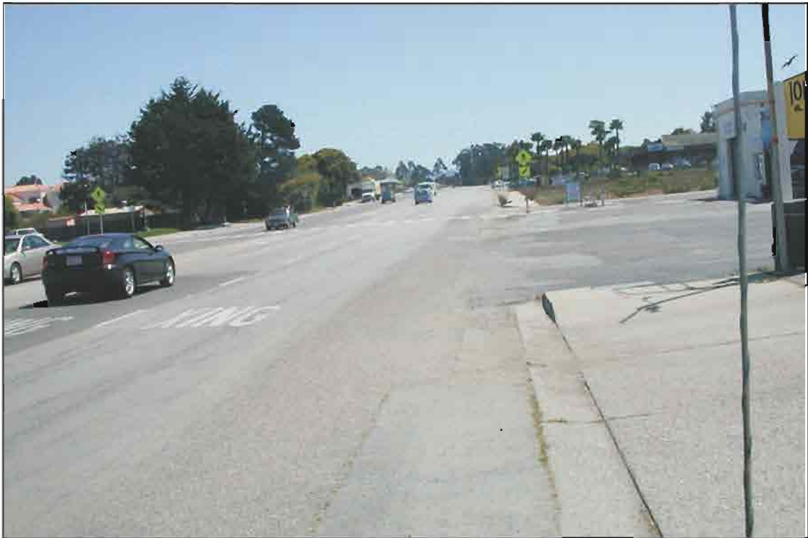
Photograph 9: View of Los Osos Valley Road right of way east of its intersection with Ninth Street, facing east.
