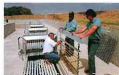
Changing an ultraviolet bulb
