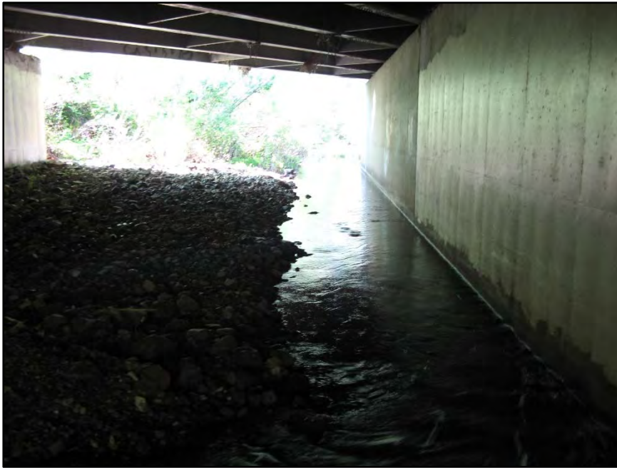
Photo 1. Looking downstream through the active “channel” of the Marsh Street Bridge.
