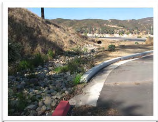
Figure 13: New storm drain
