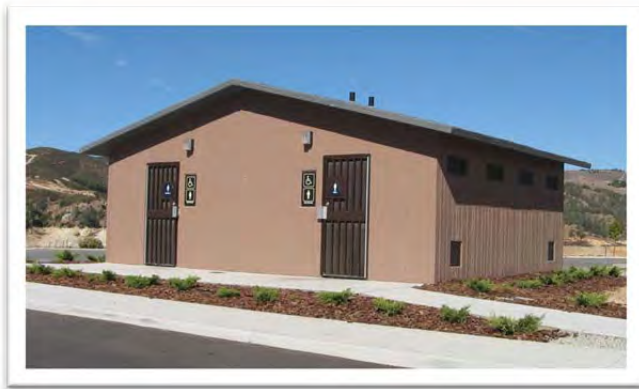
Figure 20: New flush restroom at marina
