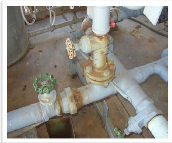
Figure 28: Old pump station (Pine Knoll)
