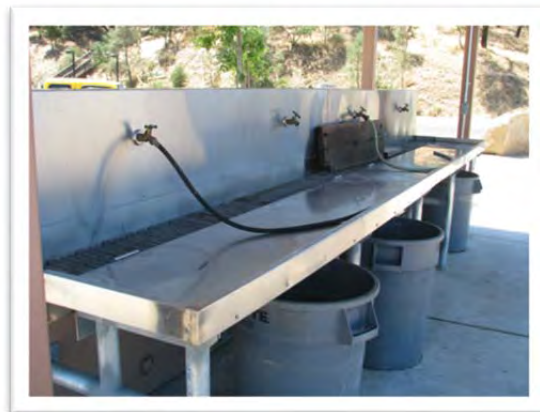
Figure 11: New fish cleaning station
