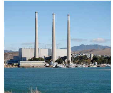
Morro Bay Power Plant
