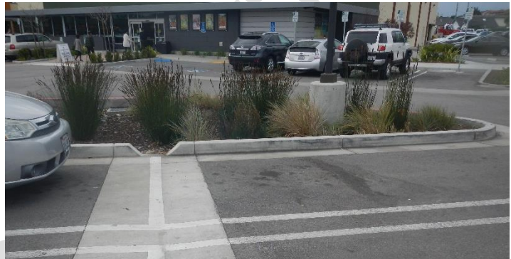
Figure 11: Recessed vegetated median with valley drain and curb cut to accept stormwater.
