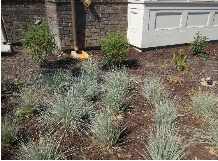
Figure 13 Downspout directed to site landscaping.
