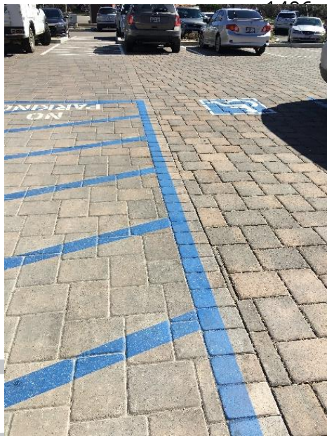
1513 Figure 18: Transition from pervious interlocking pavers to traditional pavers in ADA path of travel.
