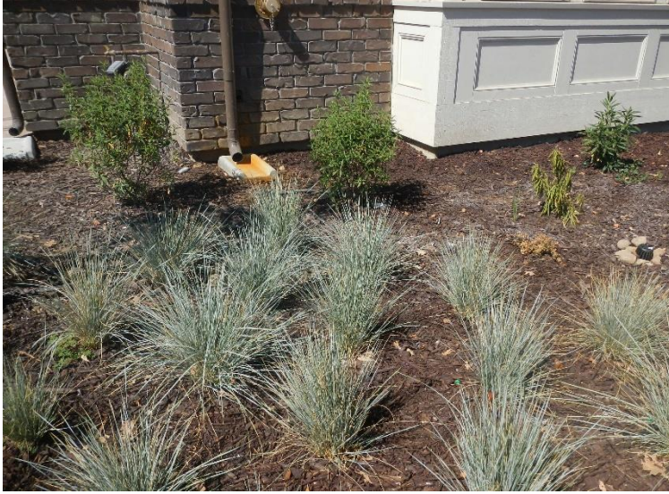
Figure 13 Downspout directed to site landscaping.
