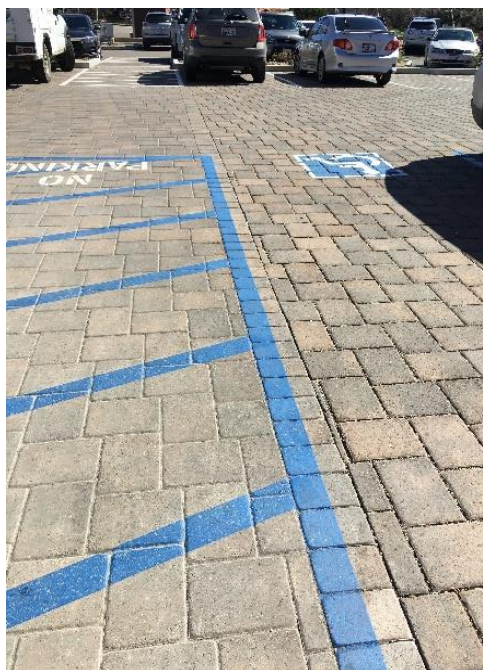
Figure 19: Transition from pervious interlocking pavers to traditional pavers in ADA path of travel.
