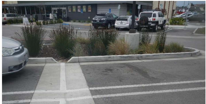
Figure 11: Recessed vegetated median with valley drain and curb cut to accept stormwater.
