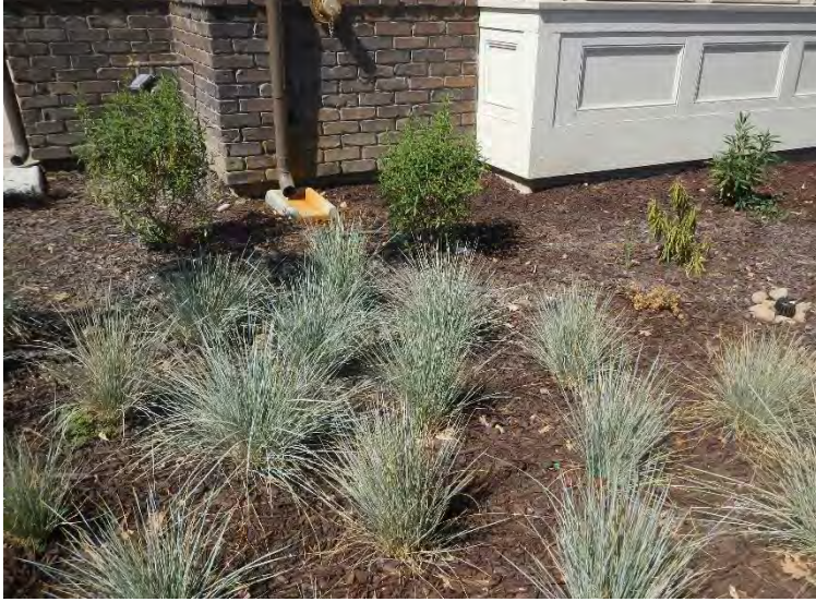
Figure 13 Downspout directed to site landscaping.
