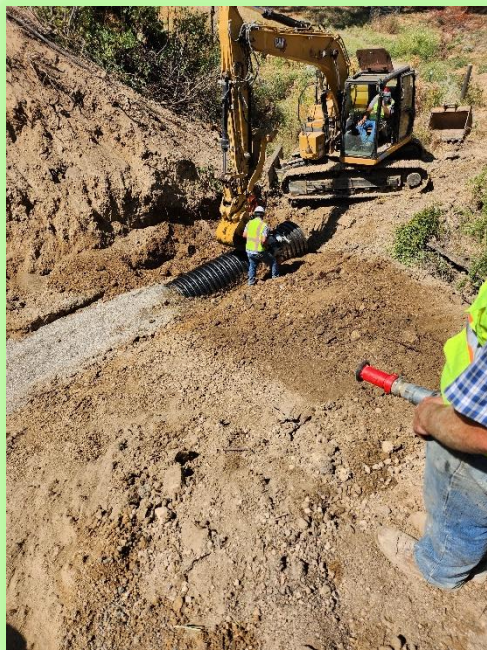
CULVERT REPLACEMENT – CHIMNEY ROCK RD, PASO ROBLES
