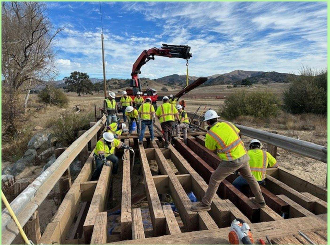
MAINTENANCE PROJECT – BRIDGE REPAIR, HUASNA ROAD BR1, MAJOR MAINTENANCE
