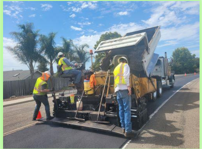
SURFACE TREATMENT – OLD OAK PARK ROAD, ARROYO GRANDE
