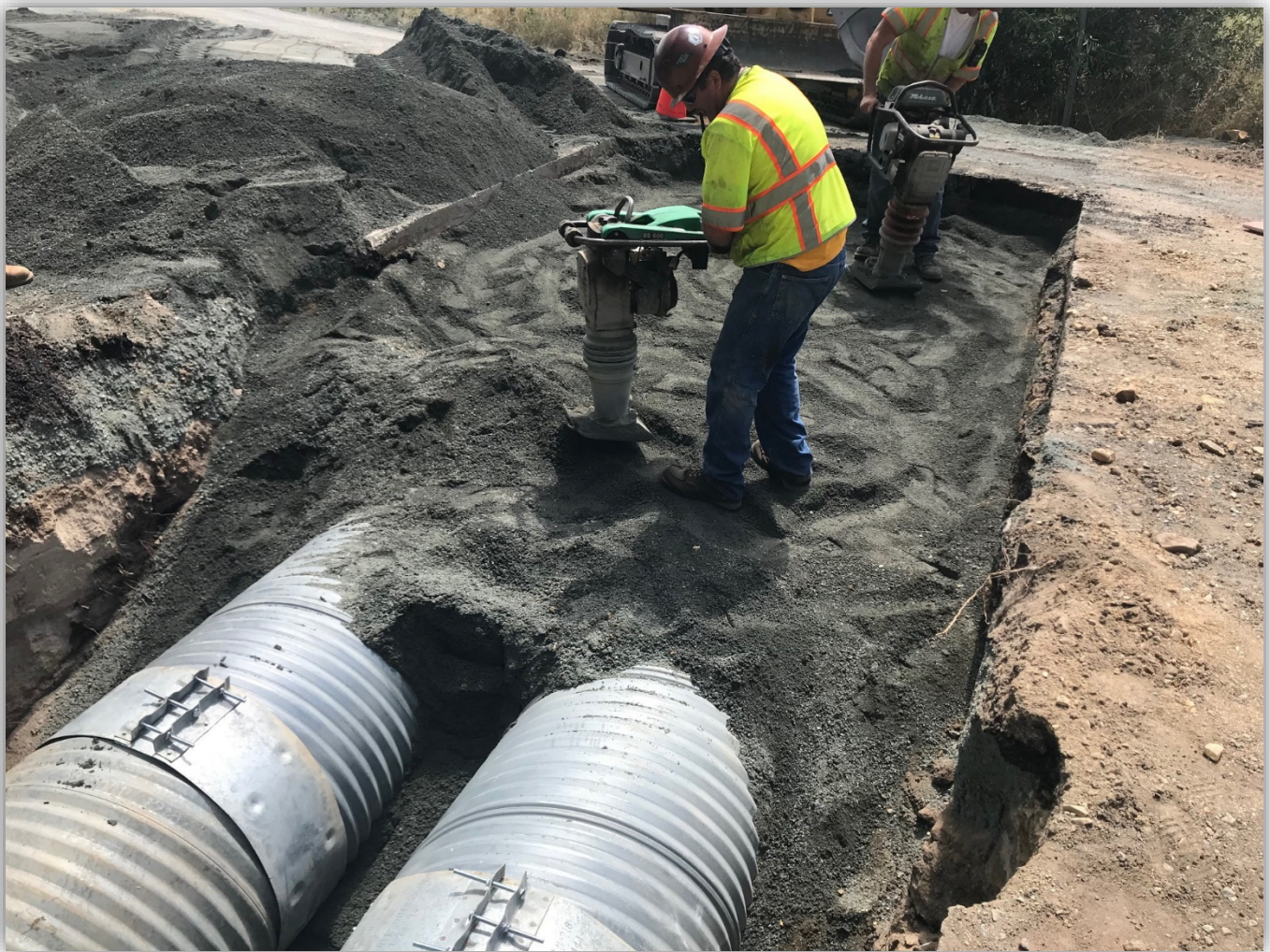
MAINTENANCE PROJECT - CULVERT REPLACEMENT, CORBETT CANYON ROAD
