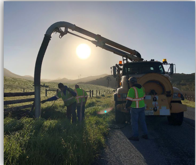
CULVERT MAINTENANCE – TURRI ROAD
