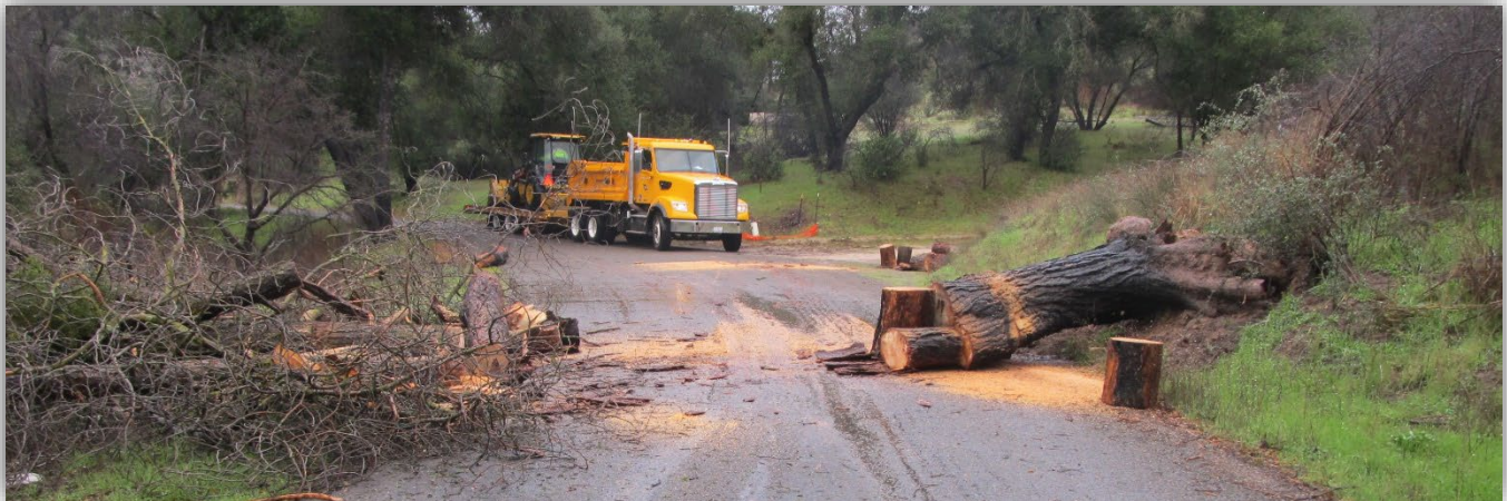
STORM RESPONSE – DOWNED TREE, LAS PILITAS ROAD
