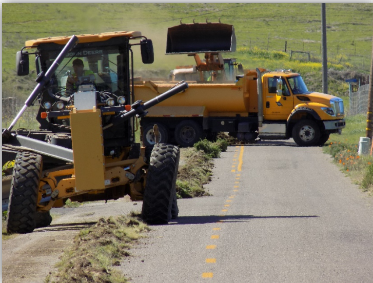
SURFACE TREATMENT PREPARATION – TORO CREEK ROAD LEFT: SHOULDER WORK, RIGHT: CRACK SEALING
