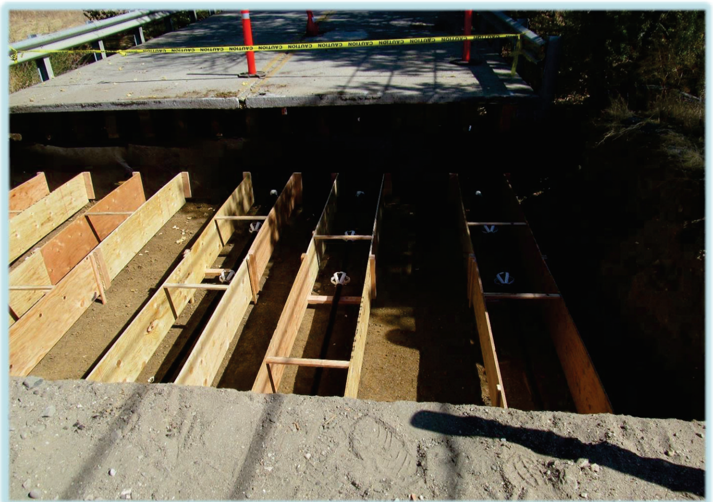
BRIDGE REPAIR - RIVER ROAD, PASO ROBLES
