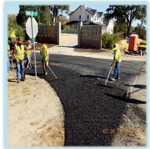
SURFACE TREATMENT – OAK FLAT ROAD, PASO ROBLES
