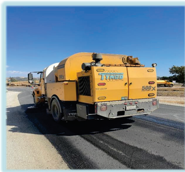
SWEEPING MAINTENANCE – THEATER DRIVE, PASO ROBLES
