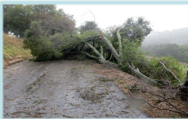
STORM RESPONSE – DOWNED TREE, PEACHY CANYON ROAD, PASO ROBLES
