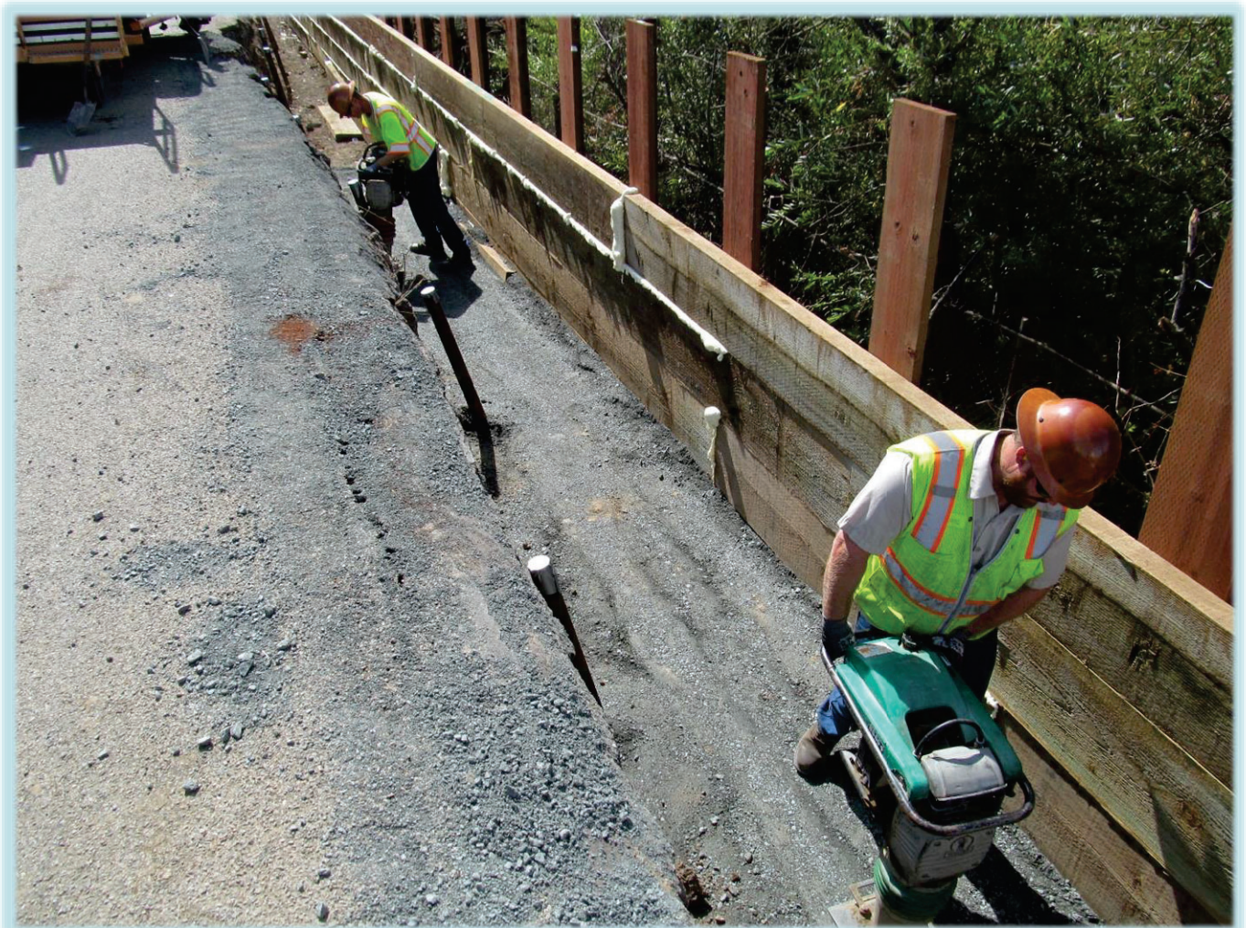
MAINTENANCE PROJECT – RETAINING WALL, HUASNA ROAD, MAJOR MAINTENANCE
