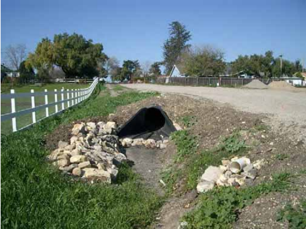
Photograph 9: Recently installed (winter 2003) Corrugated Plastic Pipe on Burton
