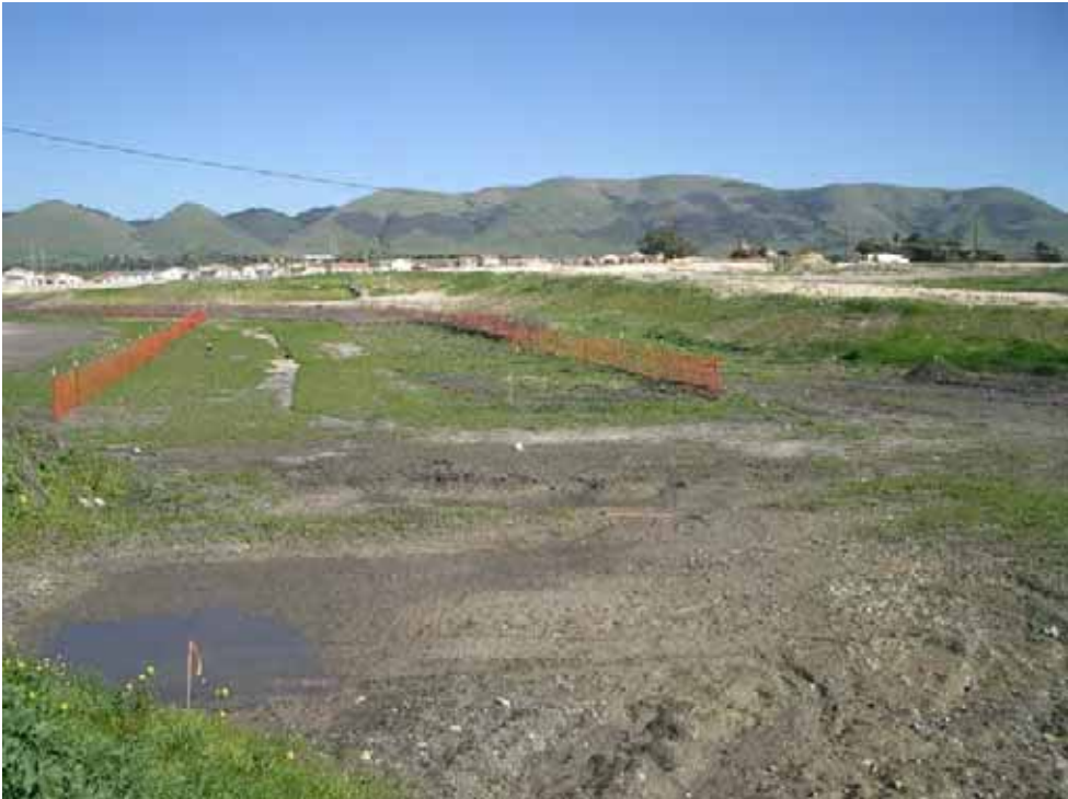
Photograph 10: Detention Basin under Construction on the Fairview Tract
