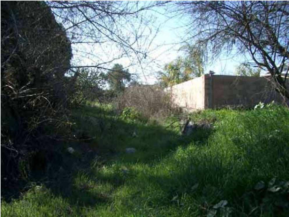
Photograph 14: Overgrown vegetation and channel encroachment on Haystack Creek
