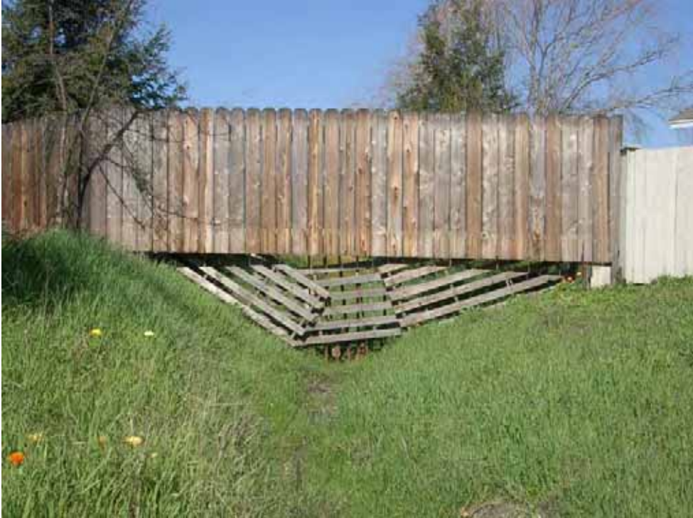
Photograph 12: Obstruction built across Hermrick Creek (typical to creeks in Olde Towne)
