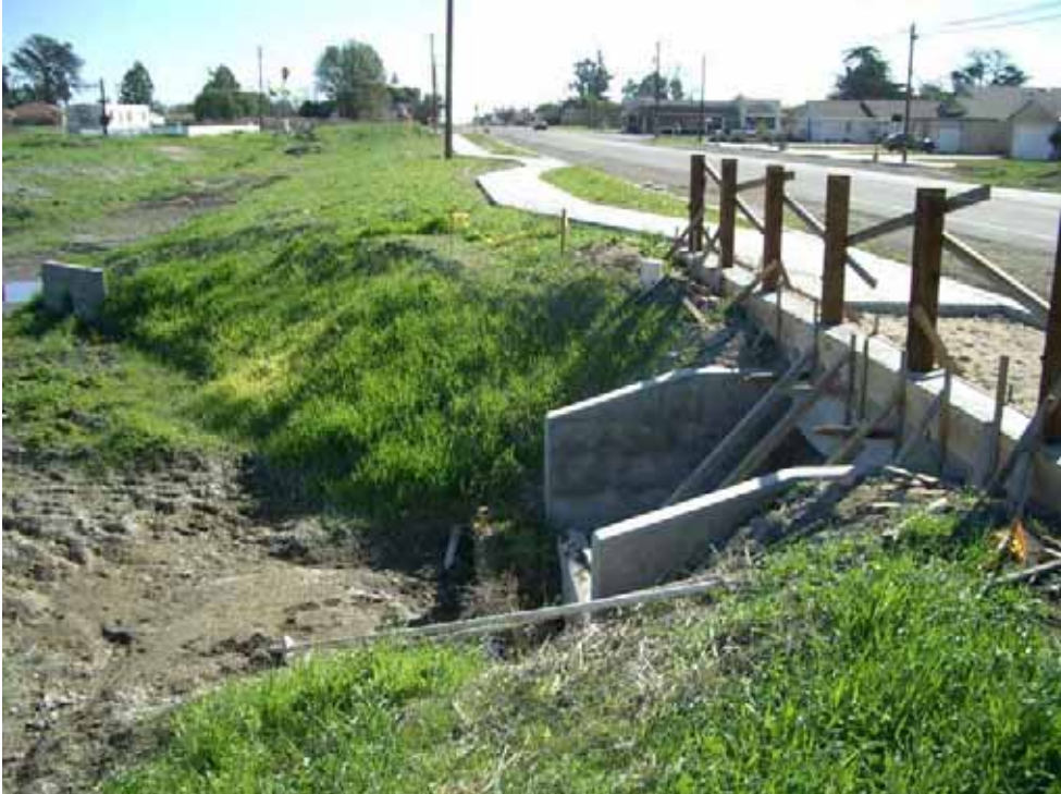
Photograph 11: Double 4'x4' Culvert at Thompson. Weir installed by Fairview Tract developer to meter flow.
