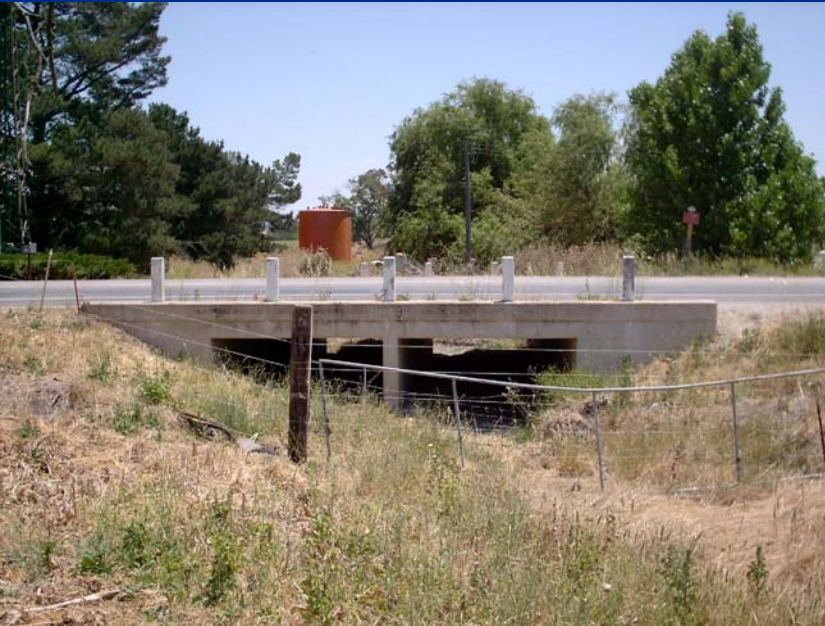
North culverts looking east
