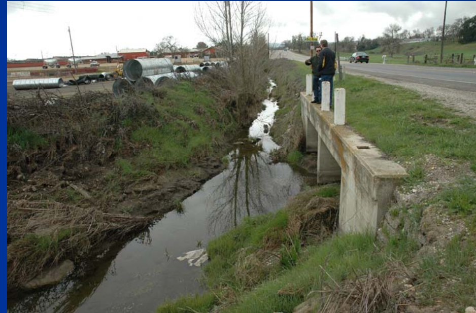
East side of Main St looking south from culvert
