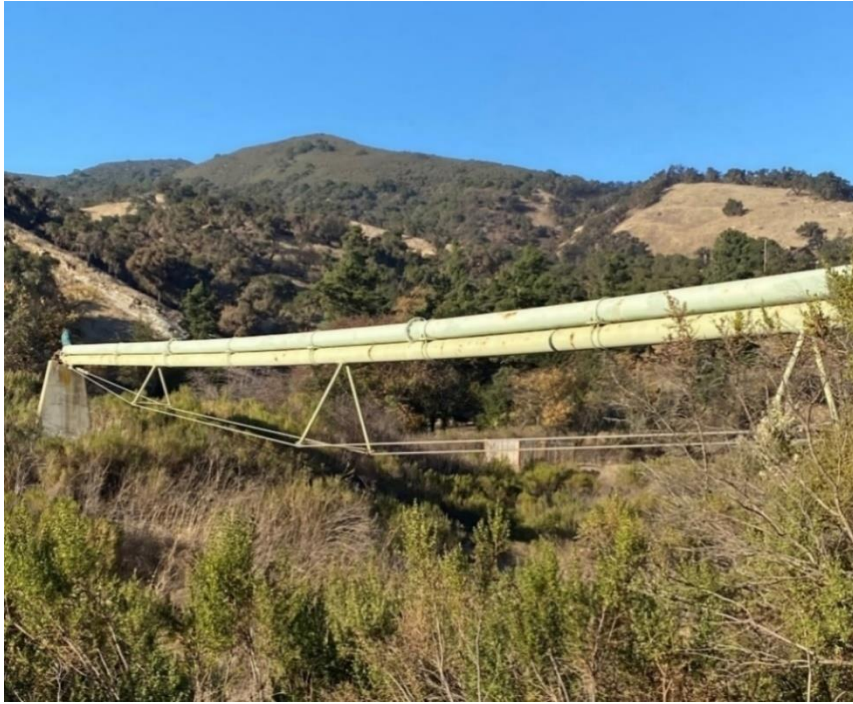
Figure 21: Sewer Force Main Over Wittenberg Creek Arm of Lopez Lake
