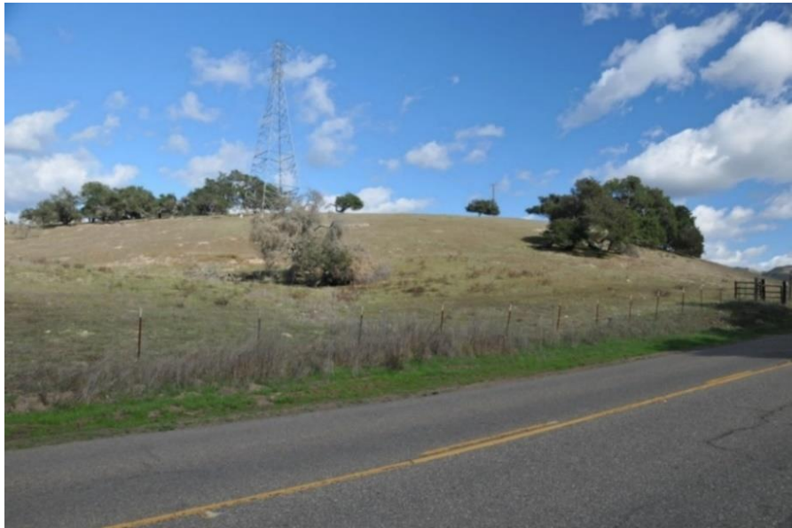
Figure 27: Terminal Reservoir Watershed Section Not Protected by Diversion Channel
