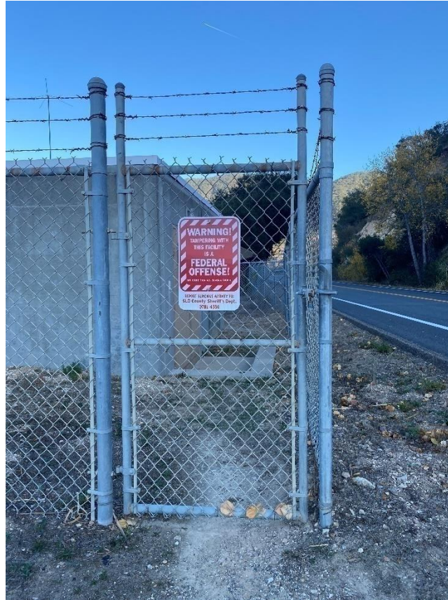
Figure 30: Locked gate at Intake structure.
