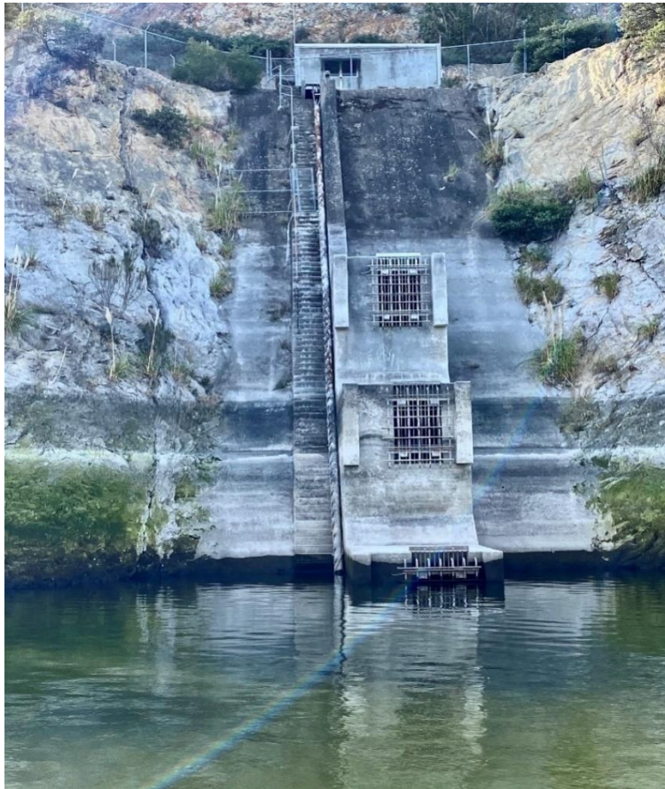
Figure 33: Lopez Lake Intake Structure
