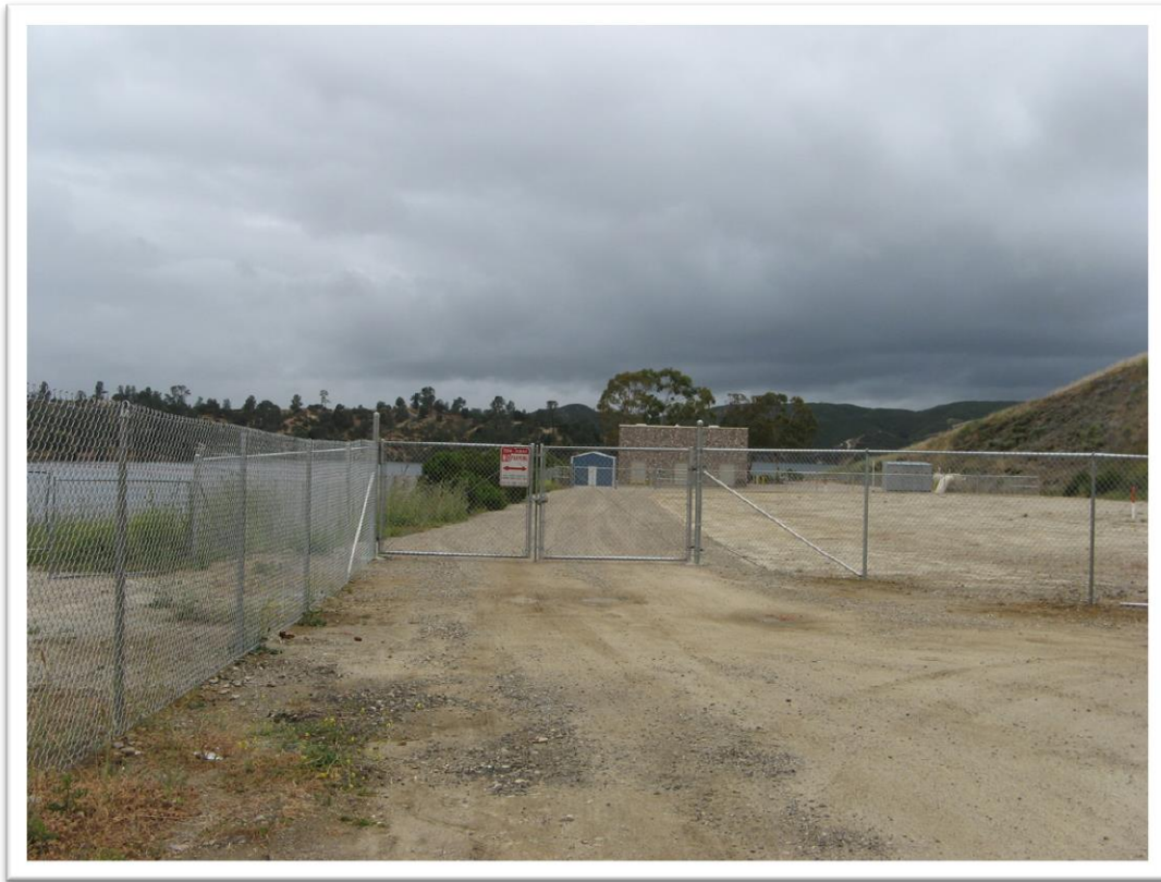
Photo: San Luis Obispo County Public Works Department Figure 38: Fencing around NWP intake pump station
