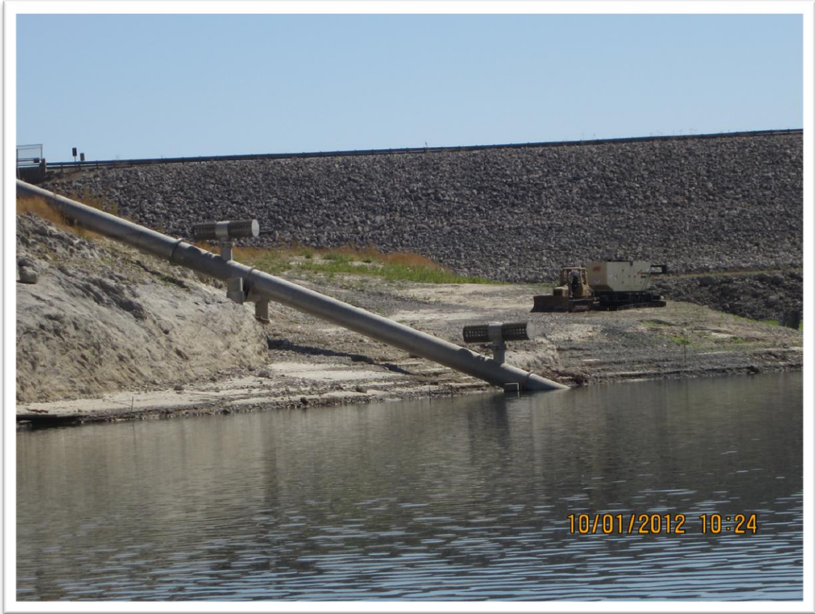
Photo: San Luis Obispo County Public Works Department Figure 34: Nacimiento Water Project intake ports
