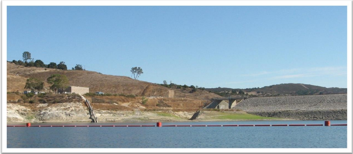
Photo: San Luis Obispo County Public Works Department Figure 37: Log boom, intake structure, and dam
