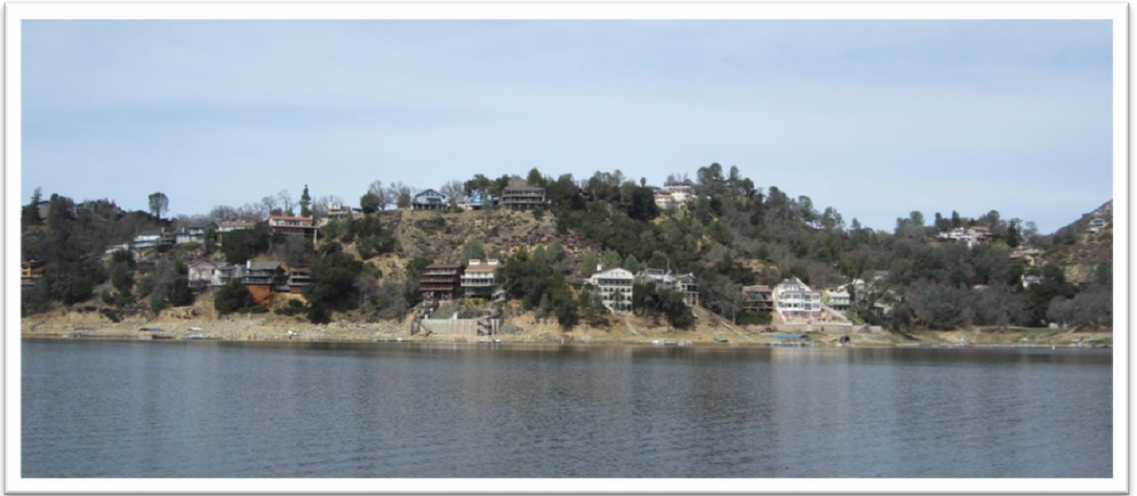
Photo: San Luis Obispo County Public Works Department Figure 55: Homes adjacent to Nacimiento Reservoir
