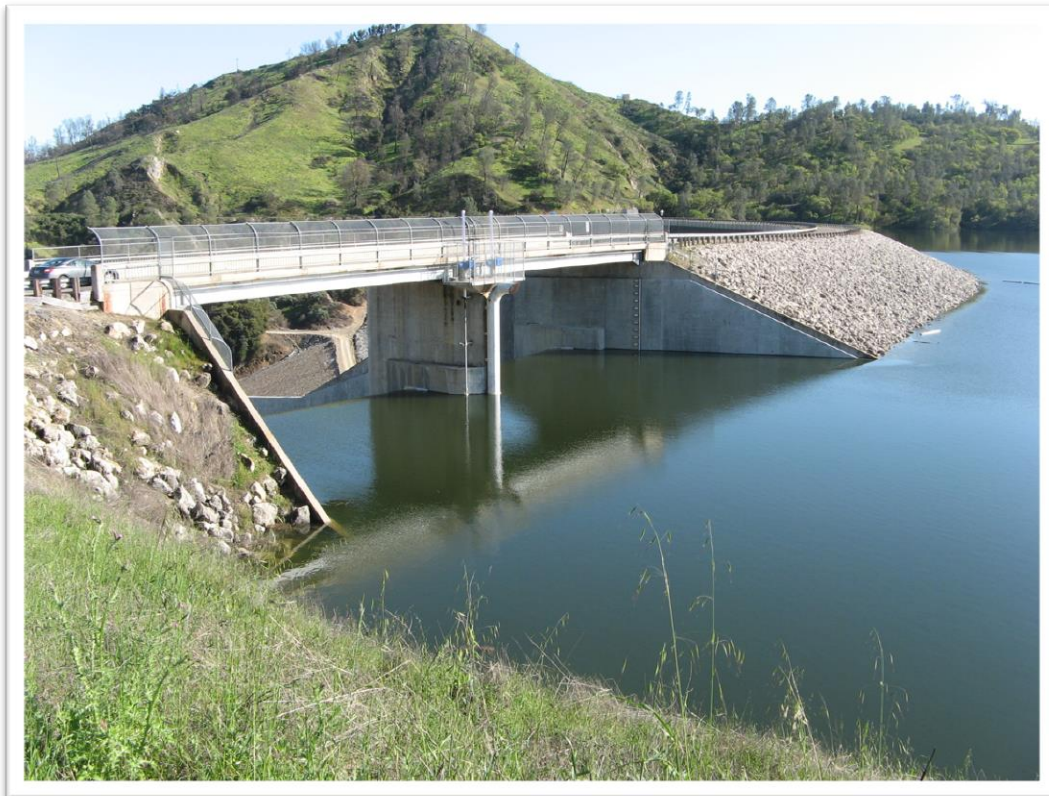
Photo: San Luis Obispo County Public Works Department Figure 32: Nacimiento Reservoir dam and spillway
