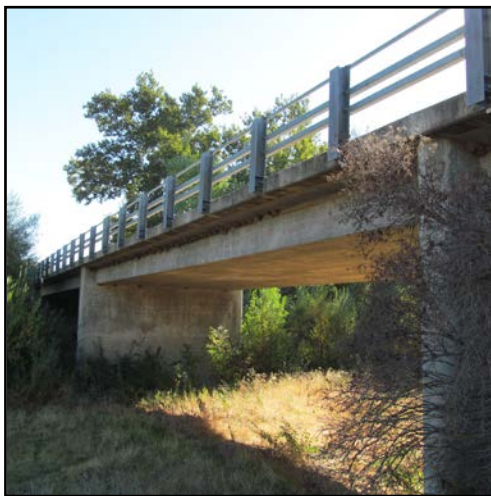
Pozo Road over the Salinas River
