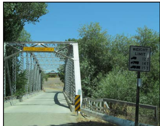
River Grove Drive over the Estrella River
