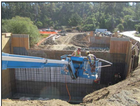
New Main Street Bridger over the Santa Rosa Creek, Cambria
