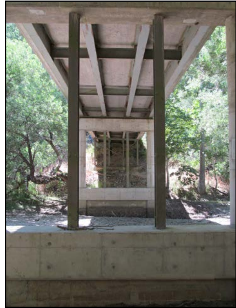
Chimney Rock Road over the Las Tablas Creek
