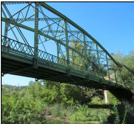
Las Pilitas Rd. Pedestrian/Bike Bridge over the Salinas River
