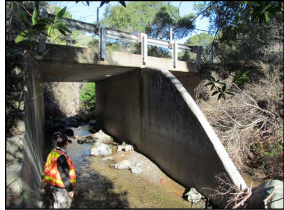
Perfumo Canyon Road over the Perfumo Canyon Creek
