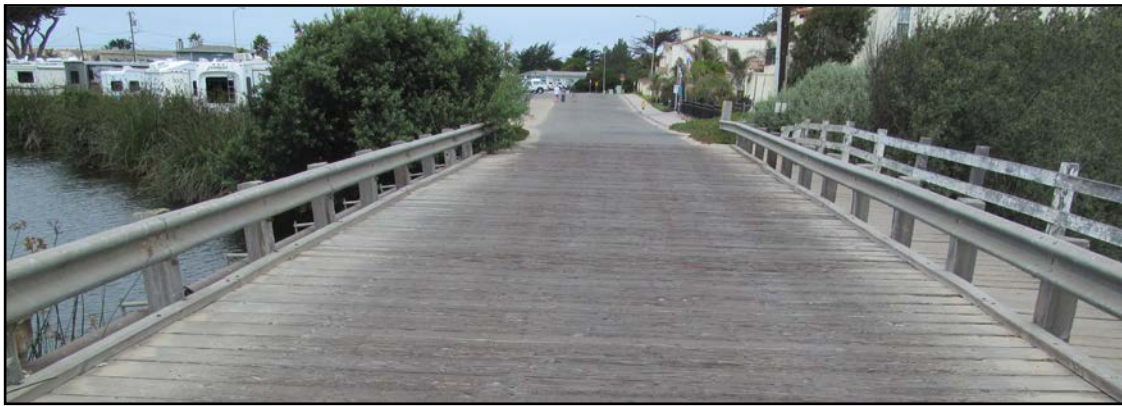
Air Park Road Bridge over the Oceano Lagoon
