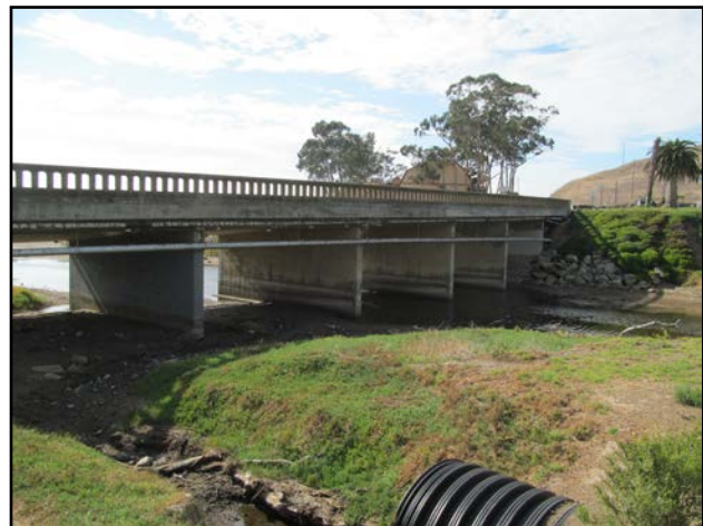
North Ocean Avenue over the Cayucos Creek
