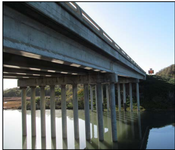
South Bay Boulevard over the Los Osos Creek
