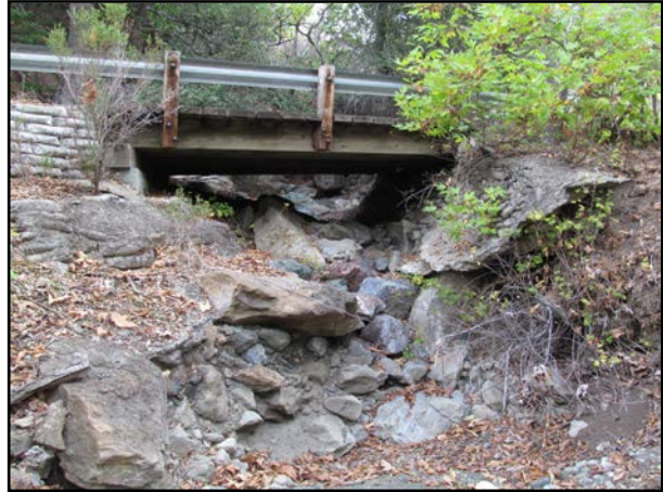
San Simeon Creel Road over the San Simeon Creek
