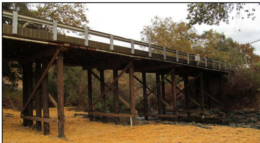
Trout Farm Road Bridge over Arroyo Grande Creek
