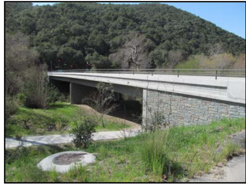
San Luis Bay Drive over the San Luis Obispo Creek
