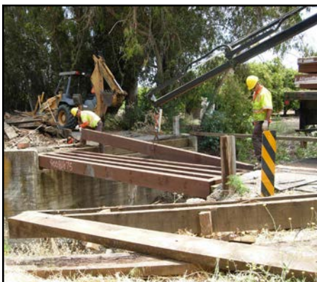
Dana Foothill Road over the Deleissigues Creek
