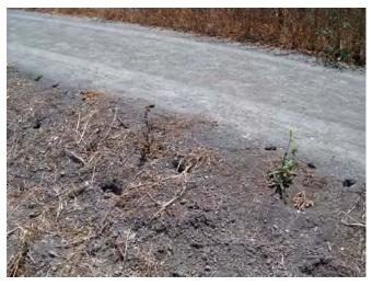
**Photo 4:** Rodent burrows observed on exterior levee slope at about Station 91+00
