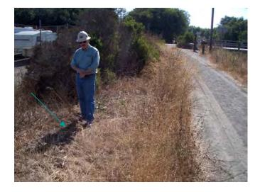
**Photo 3:** Depth of burrow approximately 4 feet at about Station 71+50 (only probe handle visible)
